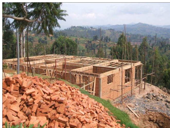
New isolation first floor (looking from the "old" NB clinic)
